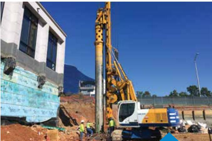
DRILLING UNDERWAY FOR SECANT PILES.
