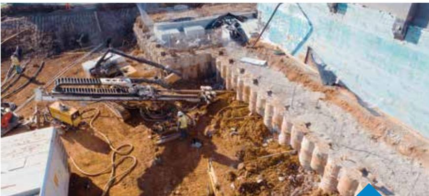
DRILLING ANCHORS THROUGH THE SECANT PILE WALL.
